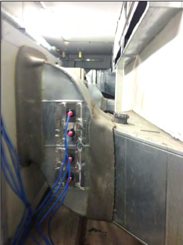
Left side of theatre 4 UV tube installation
