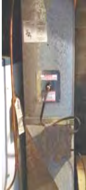
Installed UV tube in Air Duct
