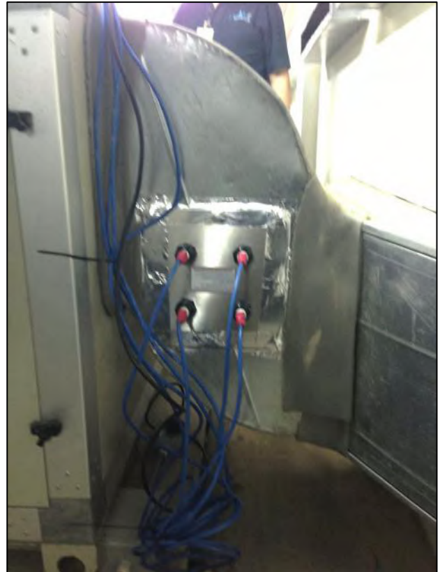
Right side of theatre 4 UV tube installation
