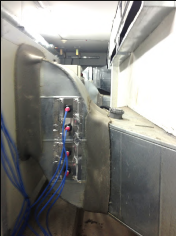
Left side of theatre 4 UV tube installation
