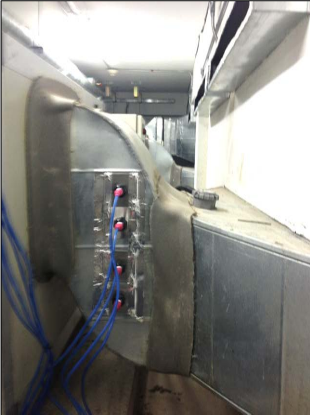
Left side of theatre 4 UV tube installation
